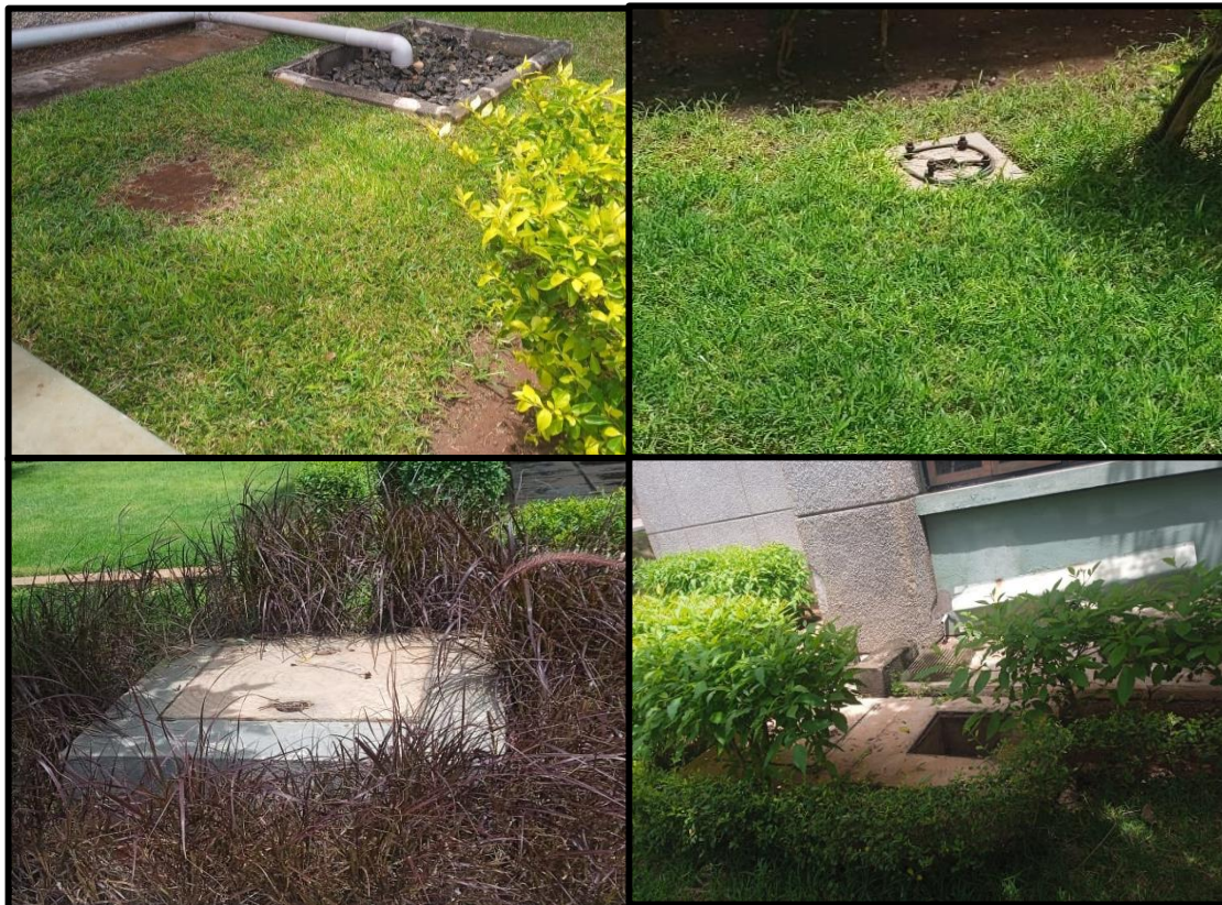
Rainwater Harvesting unit in SKASC, Coimbatore, Tamil Nadu
