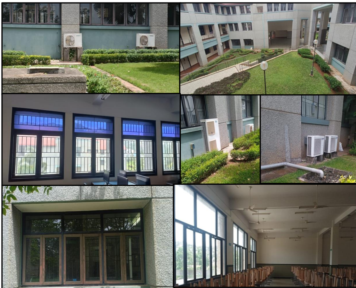
Ventilation and Exhaust system Facilities in SKASC, Coimbatore, Tamil Nadu
